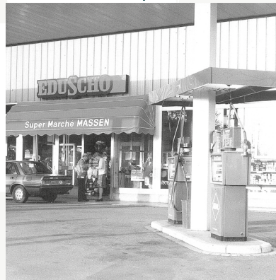
Petrol station renovation
